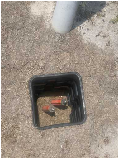
Exposed Wires-Missing Cap
